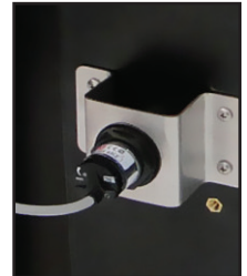
Low Water Alarm
